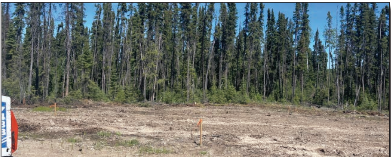
Site Prep for Kitchen Facility Next to Main Building
