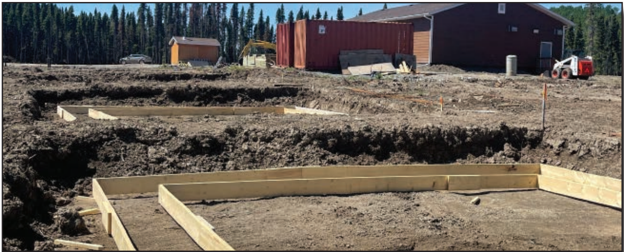
Foundations for Six Cabins
