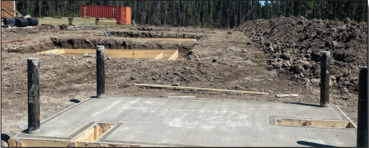
Concrete Pad for the Transformer
