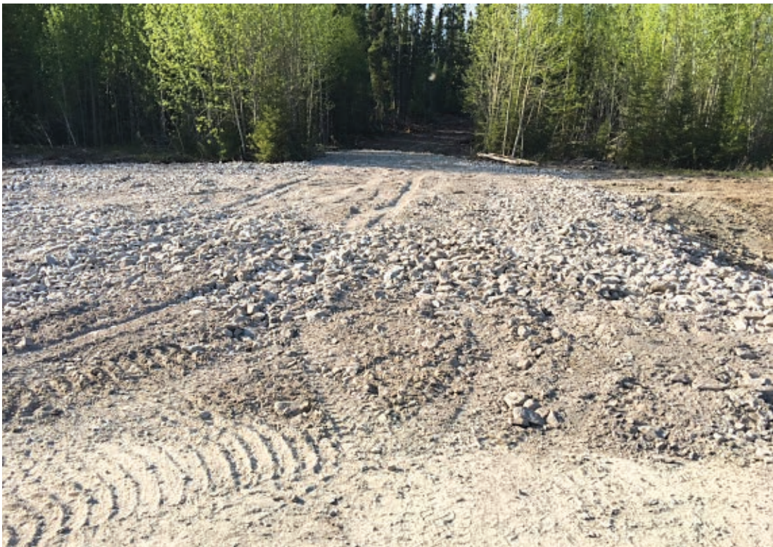
Culvert to the NNCEA culture camp completed on June 15th, 2020.
